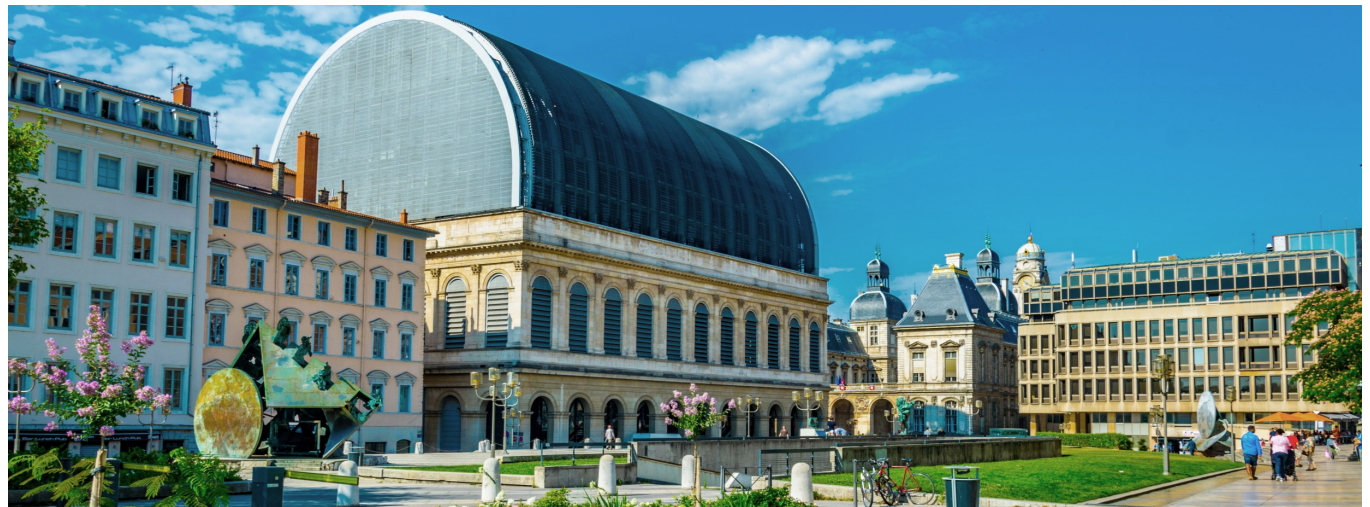
The 18-story architectural showcase Opéra National de Lyon chose a circular approach to upgrading the building's five elevators.
